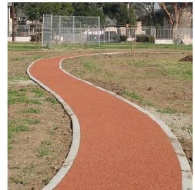
A rubber sidewalk installation, utilizing recycled post-consumer tire rubber, is part of an Urban Greening project for the Compton Unified School District (photo courtesy of Urban Greening Program and Radiant Media Solutions).
